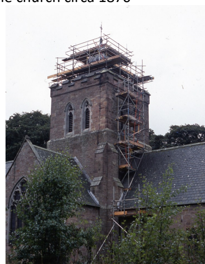
Repairs to the tower 2004
